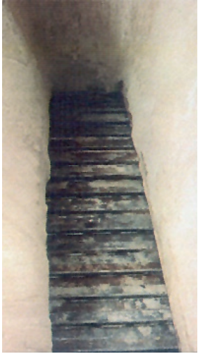
Special conveyor with reinforced plates
