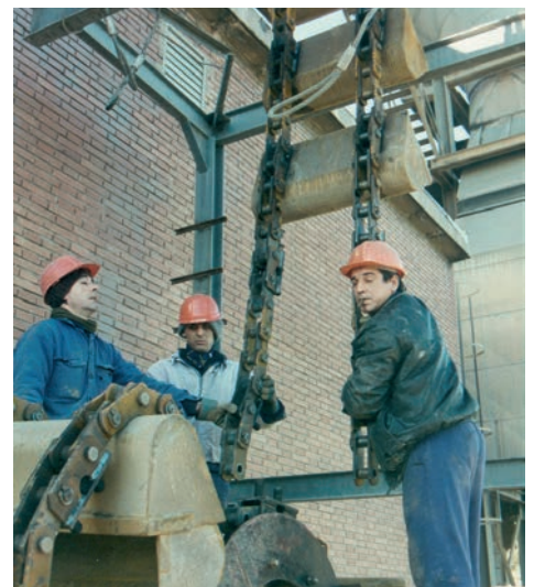
Assembly of an elevator chain
